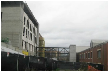
A view of the construction of the new Tioga Library Building
